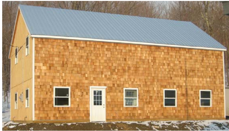
No mere sugarhouse, the maple reduction research facility at Proctor Maple Research Center in Underhill finished construction just in time for this year’s sap run.
