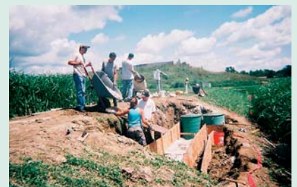
Research Assistant Professor Don Ross (upper left) assists in phosphorus filters construction at the Constructed Wetlands Center (CWC) at the Paul Miller Research Center on Spear Street. Aleksandra Drizo , research assistant professor in Plant and Soil Science and CWC project manager, states "During the first eight months of its operation, the aerated systems were capable of achieving a very high performance rate: 85-99% removal of organic matter, suspended solids, and E. coli. However, nitrogen and phosphorus removal still need to be improved."
