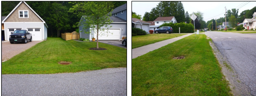
FIGURE 28. Yard drains installed within the study area, mapped as flowing into the detention pond. Note the lack of curbing. (Photos taken in July 2015.)
