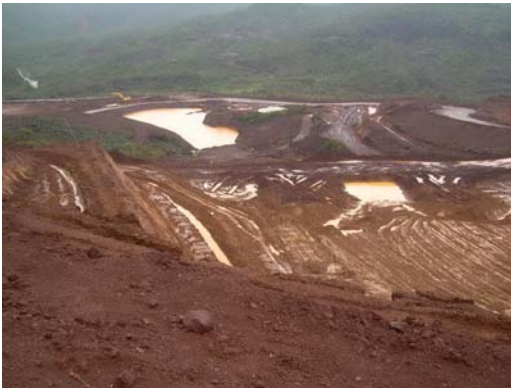
Plate 5: Construction of Processing Plant at Goro
