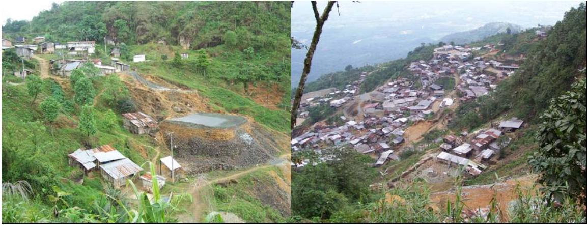
Figure 3: Processing plant and town center of Bella Rica mining concession
