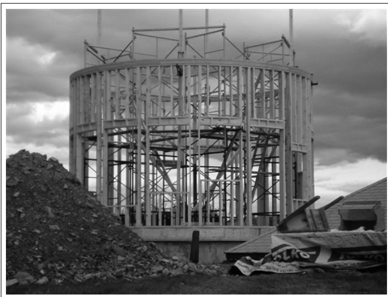
New structural framing. Courtesy of Peter Close.
