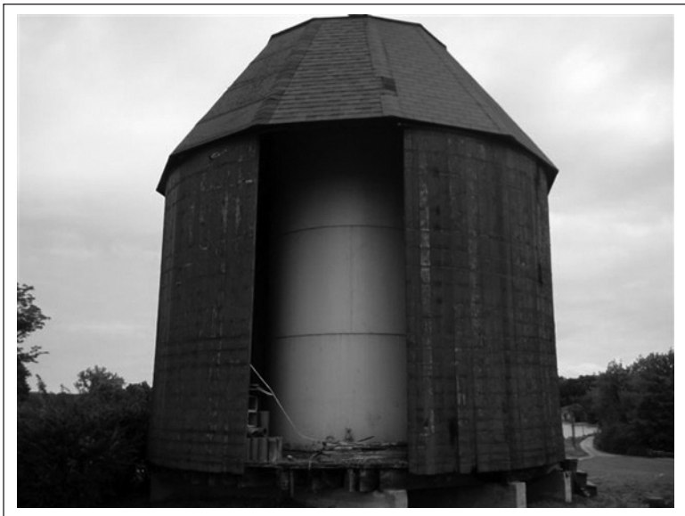
Original silo showing water cistern inside. Courtesy of Peter Close.
