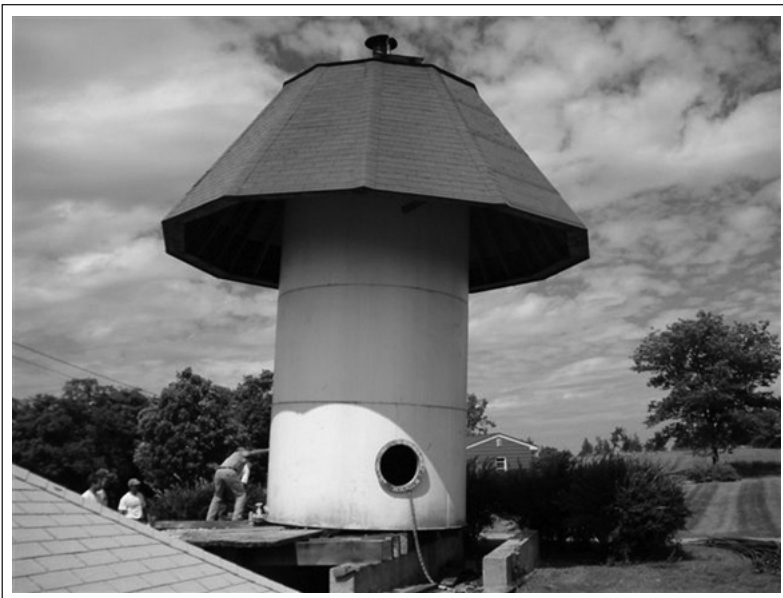
Cistern being disassembled and moved. Courtesy of Peter Close.
