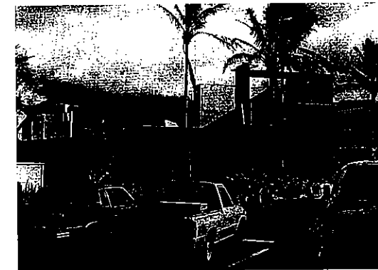
Fig. 18. Homes gutted and trees damaged by the high winds of Hurricane Iniki (1992) at Princeville, Kauai. Photograph taken one year after the storm, these homes were on a ridge fully exposed to winds that were channeled through the mountains in the distance. The channeling increased the wind speed, resulting in great damage on the lee side of the island. Photograph by Nicholas K. Coch.
