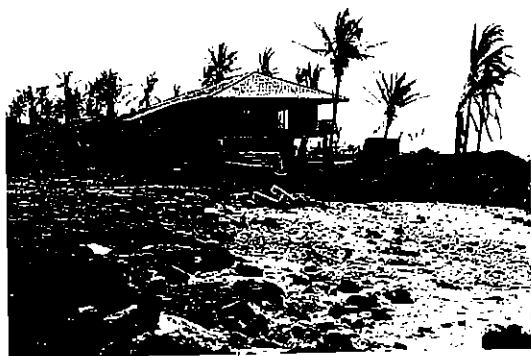
Fig. 10. Hurricane Iniki (1992) damage to homes along the Poipu coast of southern Kauai, Hawaii. Photograph taken one year after the storm. Massive waves destroyed the second story of this home. The surge and waves broke the stone wall, deeply eroded the lawn and deposited basalt boulders inland. Photograph by Nicholas K. Coch.
