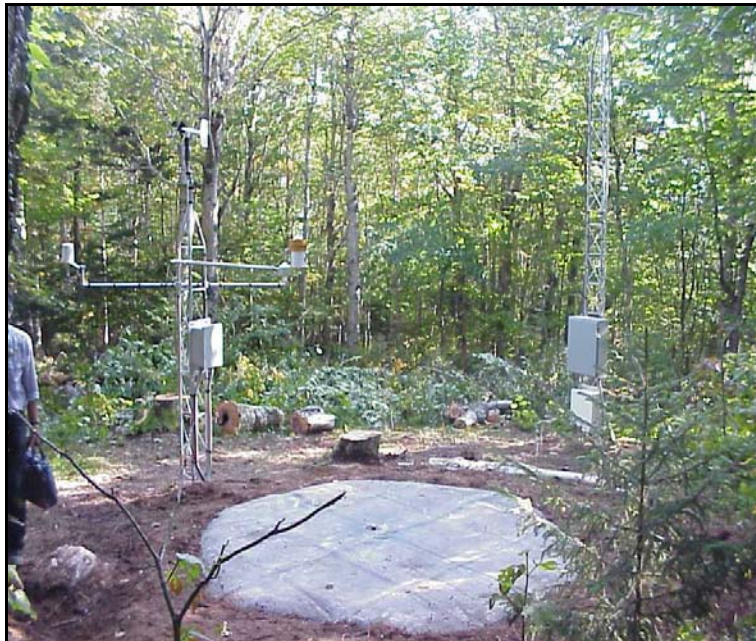
Mt. Mansfield site installation nearing completion in September 2000.
